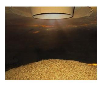
The Tunetanken wood pellet silos are of the highest quality. The silos are made of fiber-reinforced composite. A unique material that also is used for the manufacture of heavily loaded products such as wind turbines, ships, aircrafts, bridges, etc. – A material that can also be recycled.
